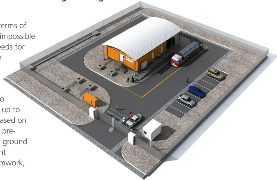
Just as with our eCentre prefabricated data centre buildings, the majority of the components are factory produced and shipped to site ready for final assembly. Using a much smaller footprint than traditional civil works, eCentre civils ensure maximum use of available site space and also allow for multi-story construction.
